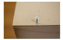
Offsetting the hole on the stage meant the screws holding the backdrop in place are not blocked.
